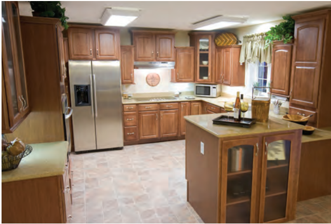
Surface mounted fixtures providing downward light coupled with an over-sink task light and under-cabinet lights. (Photo courtesy of Laurence Weinstein)
