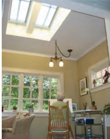
The balanced daylight in this room is ideal for painting and relaxing. Indirect lighting reflected from the skylight well provides general illumination for the space as daylight dims. (Photo credit: Eunice Noell-Waggoner)
