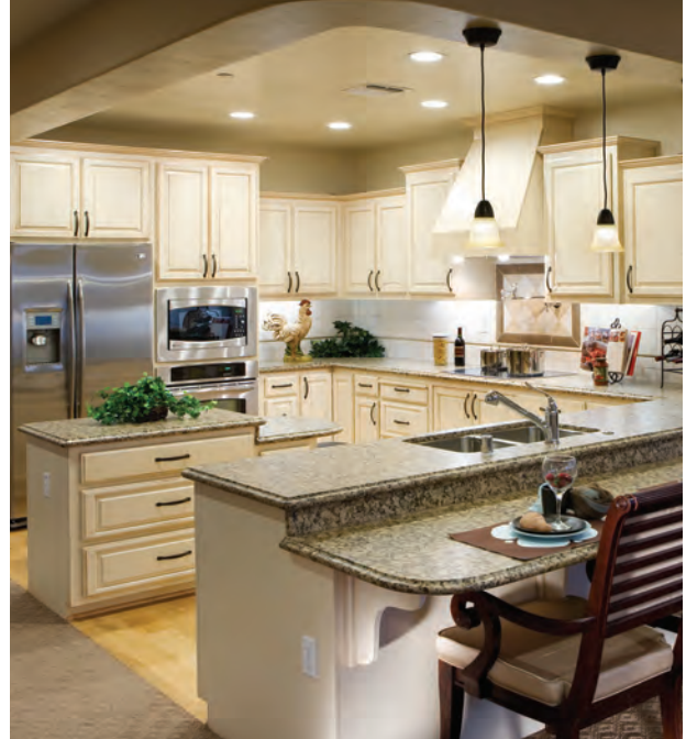
This kitchen utilizes slim surface-mounted ceiling LED fixtures, pendant fixtures with diffusing glass to cut glare, and under-cabinet lighting, which serves as good task lighting at the counters. Light-colored matte surfaces also help to provide glare-free reflected light. (Photo courtesy of Laurence Weinstein)
