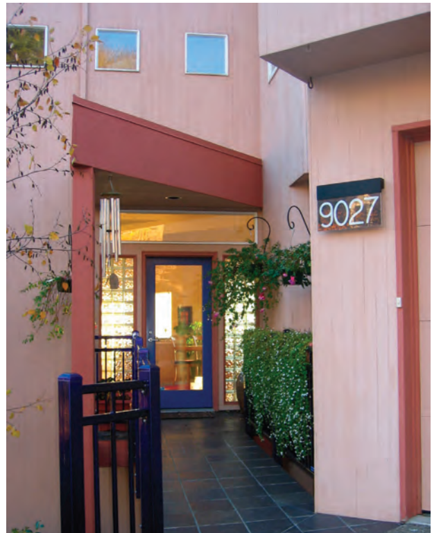
The high contrast of the white house numbers against a black background makes them easy to read during the day. At night, a photocell turns on an integrated light source illuminating the numbers to increase their visibility when it is dark.
