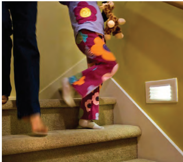
LEFT: An LED channel with a motion sensor and a grazing light with an optical lens was added to light the stairway and specifically the stair treads. The wall color has a high light reflectance value (LRV 86) so that the light from the one fixture illuminates the space. The contrast of the darker carpet against the white stair skirting helps to define the steps. RIGHT: Step lights spaced frequently along the stairway and landing are another good option to light the treads (Right photo courtesy of Eunice Noell-Waggoner; left photo courtesy of Laurence Weinstein)
