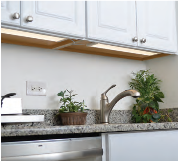
LED fixtures installed under upper cabinets.
