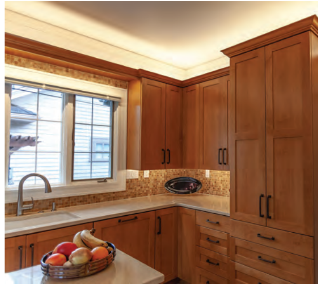
Indirect LED strip lighting provides a diffused ambient light to the space, while additional task lighting is provided over the sink and under the cabinet to light the work surface. Daylight from two directions balances the daylight in the space. Ceiling, walls and countertop are light colored. (Photo courtesy of Yadira Pagan Fuentes)
