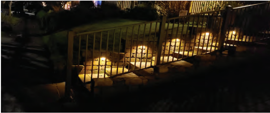
Wall mounted step lights provide light across the tread. The light source is well concealed to prevent glare. (Photo courtesy of Eunice Noell-Waggoner)
